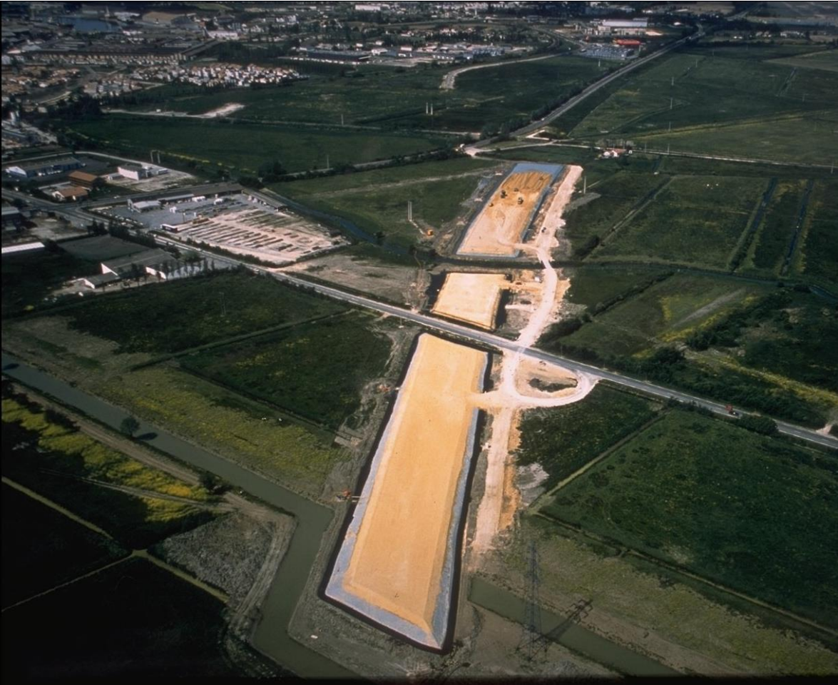
Tonnay Charente swamp area with 2 m high fill on membrane
