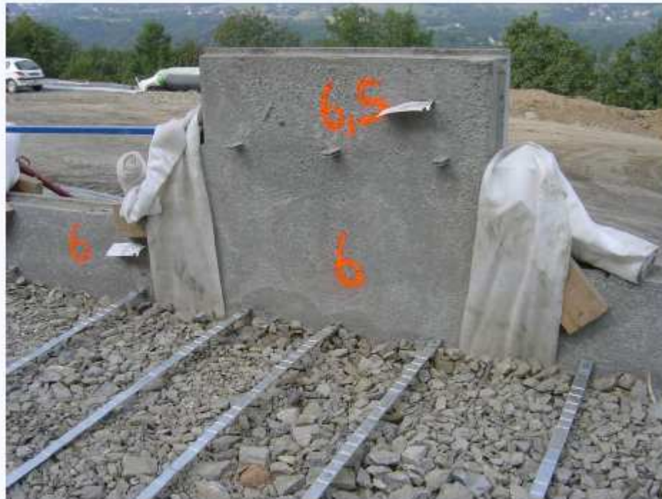
Concrete Facing with Metallic Strips
