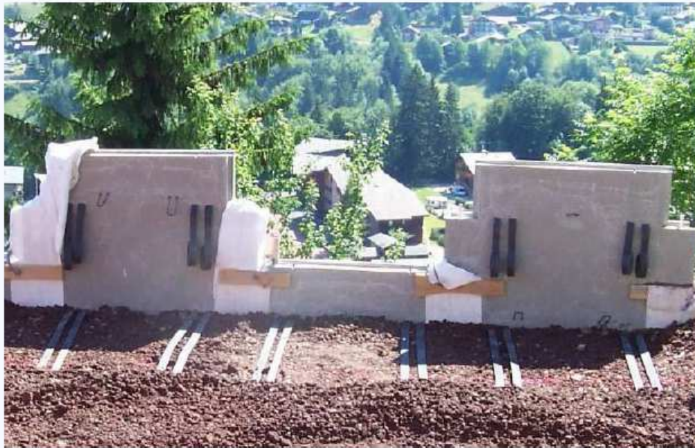
Concrete Facing with Geosynthetic Strips or Grids
