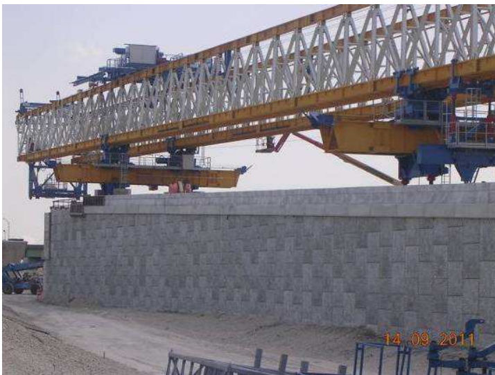
Bridge launching gantry - USA
