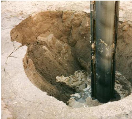
Figure 6: Crater due to execution
