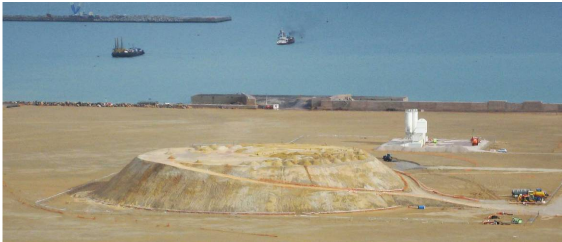
Photo 2: Completed Preload of Tank Nr 1
