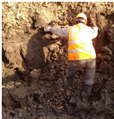
Photo 4 : Excavated stone column 2 weeks after construction
