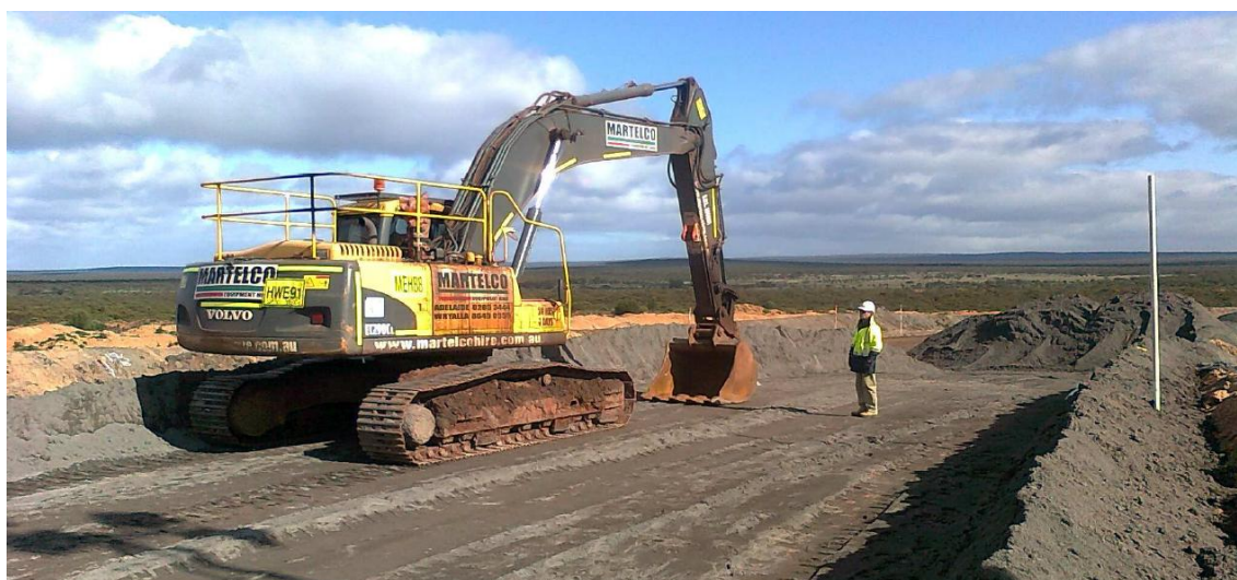
Photo 2: Test pad construction showing excavator used.
