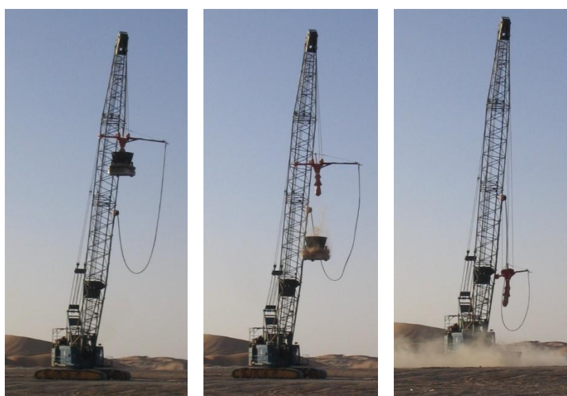
Figure 3: MARS automated drop and grab system
