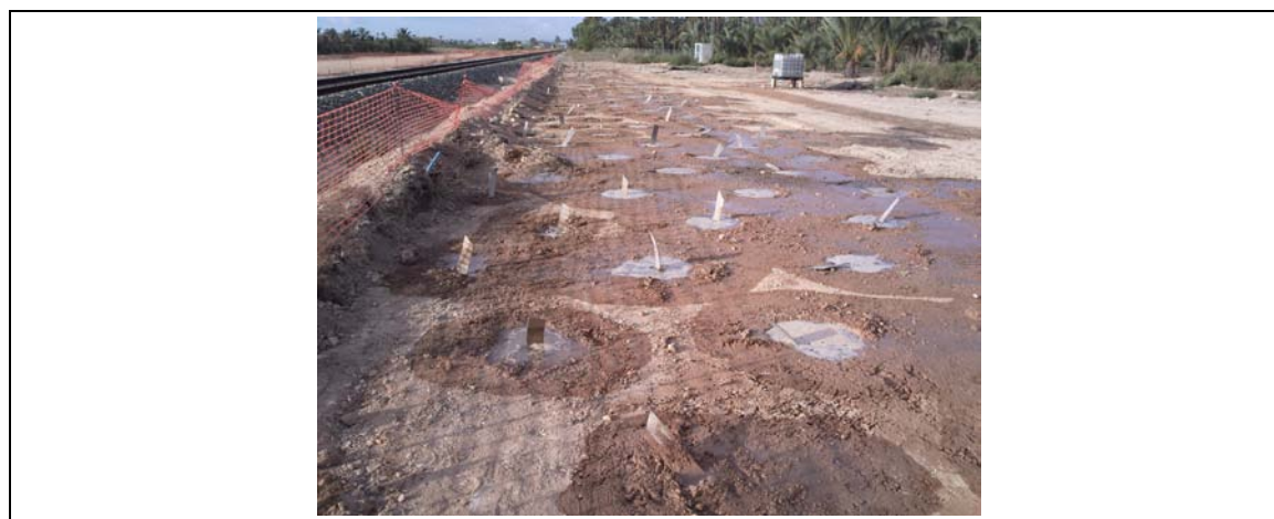
Photo1: Treatment by vertical drains.
