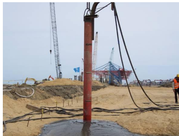
Photo 2: Operation of vibro-compaction in action
