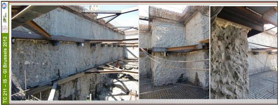
Figure 19: Views of the excavation works, with no water inflow, and details of the compatibility of the CSM panels with the internal structures.
