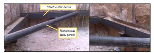
Figure 11: Detail of the steel waler beams connected to the pipe struts.
