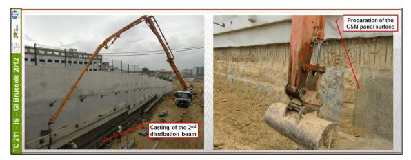
Figure 14: Views of the excavation works.
