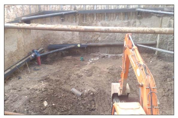
Figure 12: View of the work after the execution of the second level of struts.
