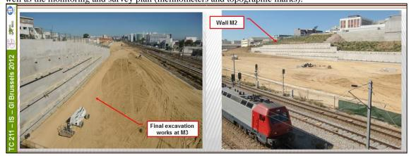
Figure 15: Views of the walls after the conclusion of the excavation works.
