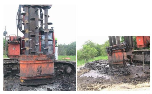
Figure 1: The triple auger system used in the field trials to install the PRB walls, low permeability wall sections and individual S/S sections
