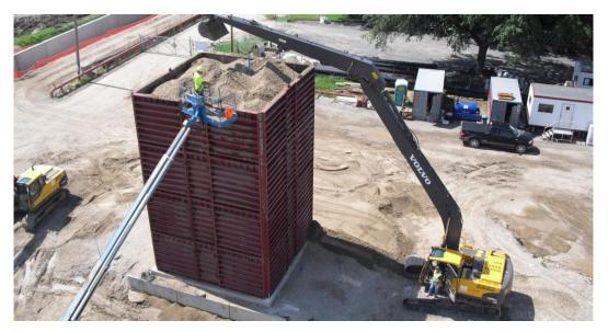
Figure 8: Picture of the construction of the Load Test Area (Form Work)
