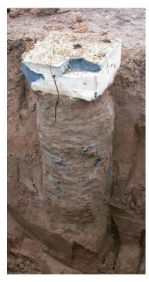
Figure 3: Excavation of column P2
