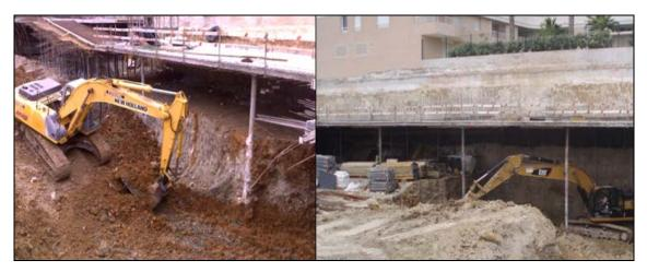
Figure 10: Views of the work during the execution of the second level of excavation.
