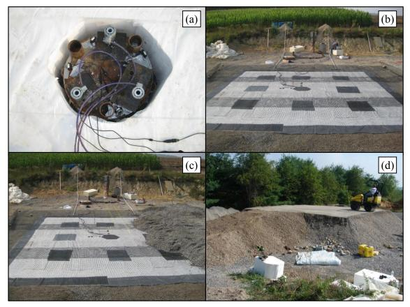
Figure 6: a) load cells and webcams in central column, b) first layer of geogrid over the geofoam and columns, c) placement of the first fill layer, d) compaction of fill on an embankment nearing completion.
