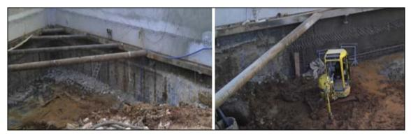
Figure 12: Partial views of the steel pipe struts.
