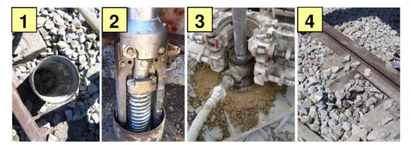
Photo 2: installation procedure for columns under existing tracks.
