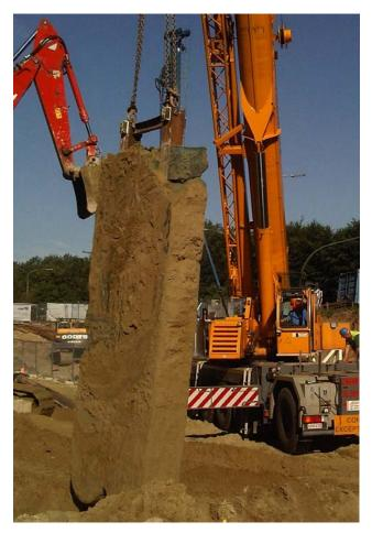
Figure 3: Excavation of an in situ executed CSM panel (Lameire Funderingstechnieken n. v.)
