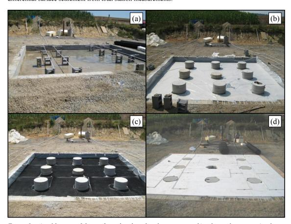
Figure 5: a) calibration of the geofoam dissolver distribution system, b) column placement, c) columns with geonet placed at the base of the mat foundation, and d) working platform for embankment construction after placement of geofoam.
