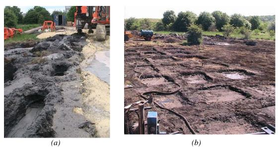
Figure 8: The completed individual sections (a) triple auger S/S sections and (b) the ALLU mass stabilisation sections.
