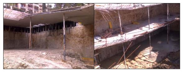
Figure 11: View of the work during the second level of excavation (on the left) and after the execution of the second level of slab bands (on the right).
