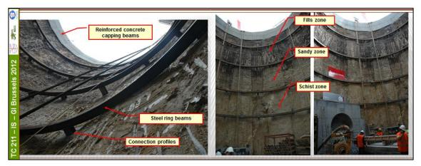
Figure 8: Views from the inside of the right bank shaft after excavation.
