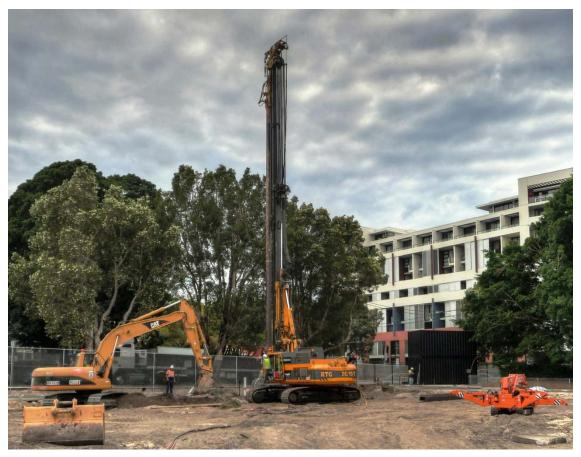
Photo 5: RTG RG 19 T and excavator for pre-excavation and backflow handling
