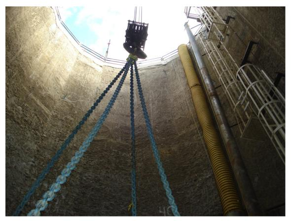
Photo 7: Excavated shaft L, excavation depth about 22 m
