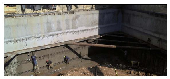
Figure 8: Partial view of the retaining wall with the steel waler beams, the internal struts and the concrete wall.
