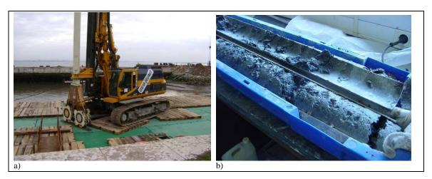
Photo 1: a) CSM RG 19 rig; b) core samples from test panels
