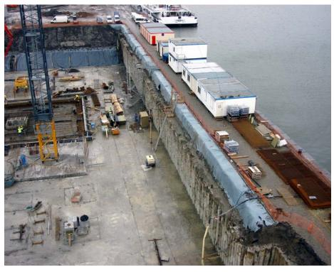
Figure 1: SMW with ground and water retaining functions
