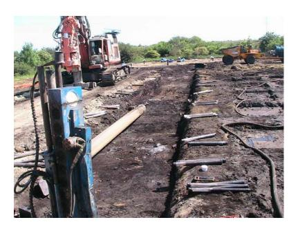
Figure 11. Window sampling from the individual triple auger S/S sections
