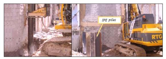
Figure 10: View of the execution of a CSM panel (on the left) and installation of the IPE piles (on the right).
