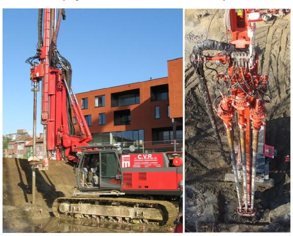
Figure 3: CVR C-mix® machine and its Triple version
