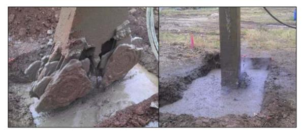
Figure 9: Execution of a CSM panel.
