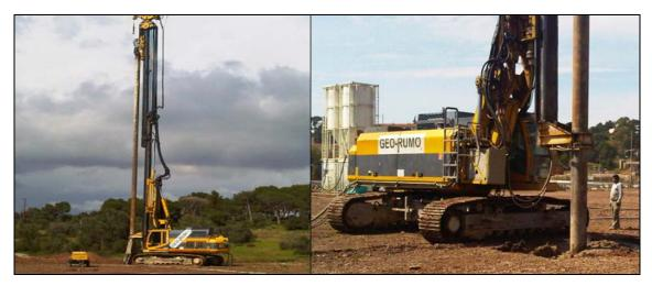
Figure 8: Equipment to the application of CSM technology.
