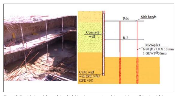
Figure 5: Partial view of the work (on the left) and cross-section of the retaining wall (on the right).
