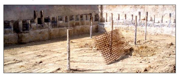
Figure 9: Foundation micropiles to the temporary support of the slab bands.
