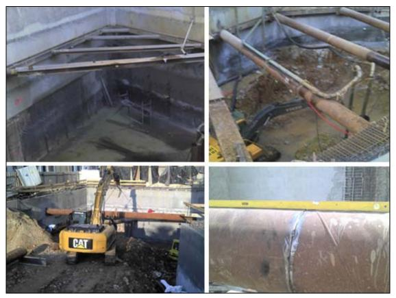
Figure 14: Different views of the work and a detail of a pipe strut.
