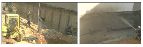
Figure 13: Execution of the concrete wall.
