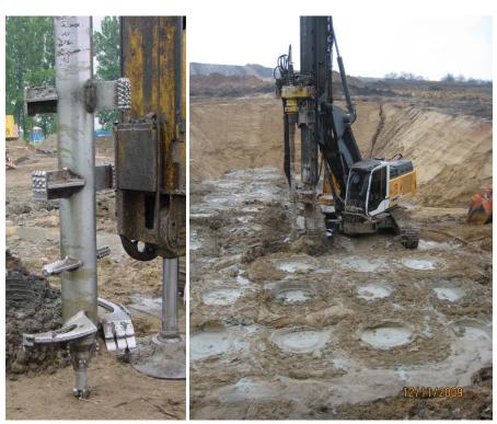
Photo 2: DSM Mixing tool with one shaft and four blades (left) and rig with single shaft mixing tool (right) (property of Keller Grundbau GmbH)
