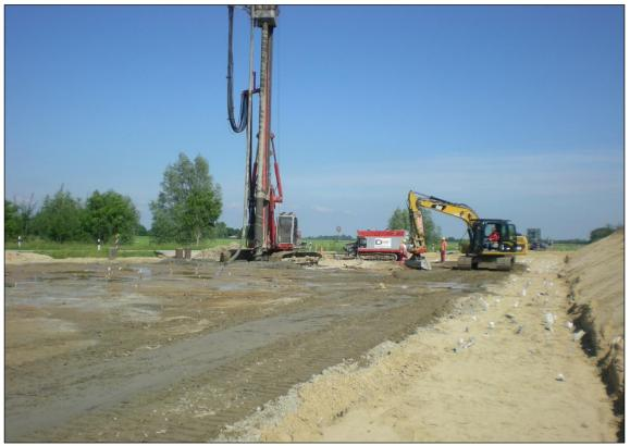
Photo 2: installation of CMC combined with vertical drains with water on the platform
