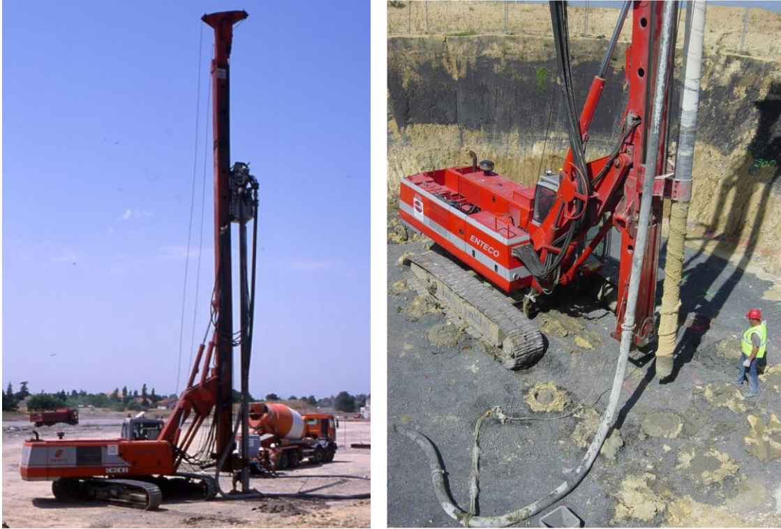
Fig. 2. Installation of CMC columns in two projects in France
