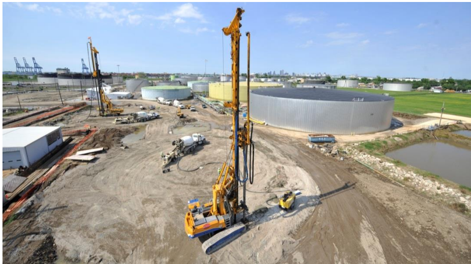
Fig. 24. Installation of 34 m long CMC
