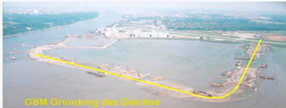
Lot 1 : Dyke construction
