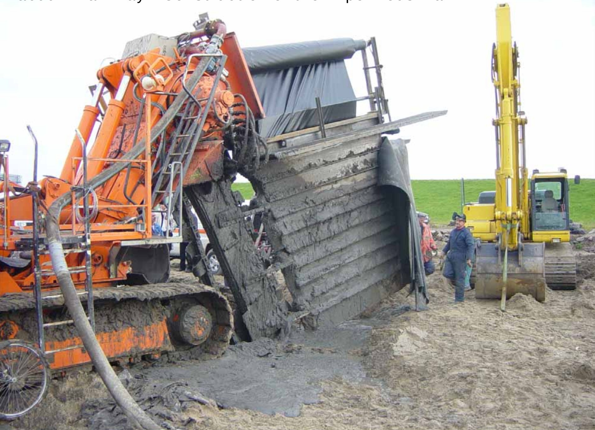
Vacuum Taxiway – Construction of the impervious wall
