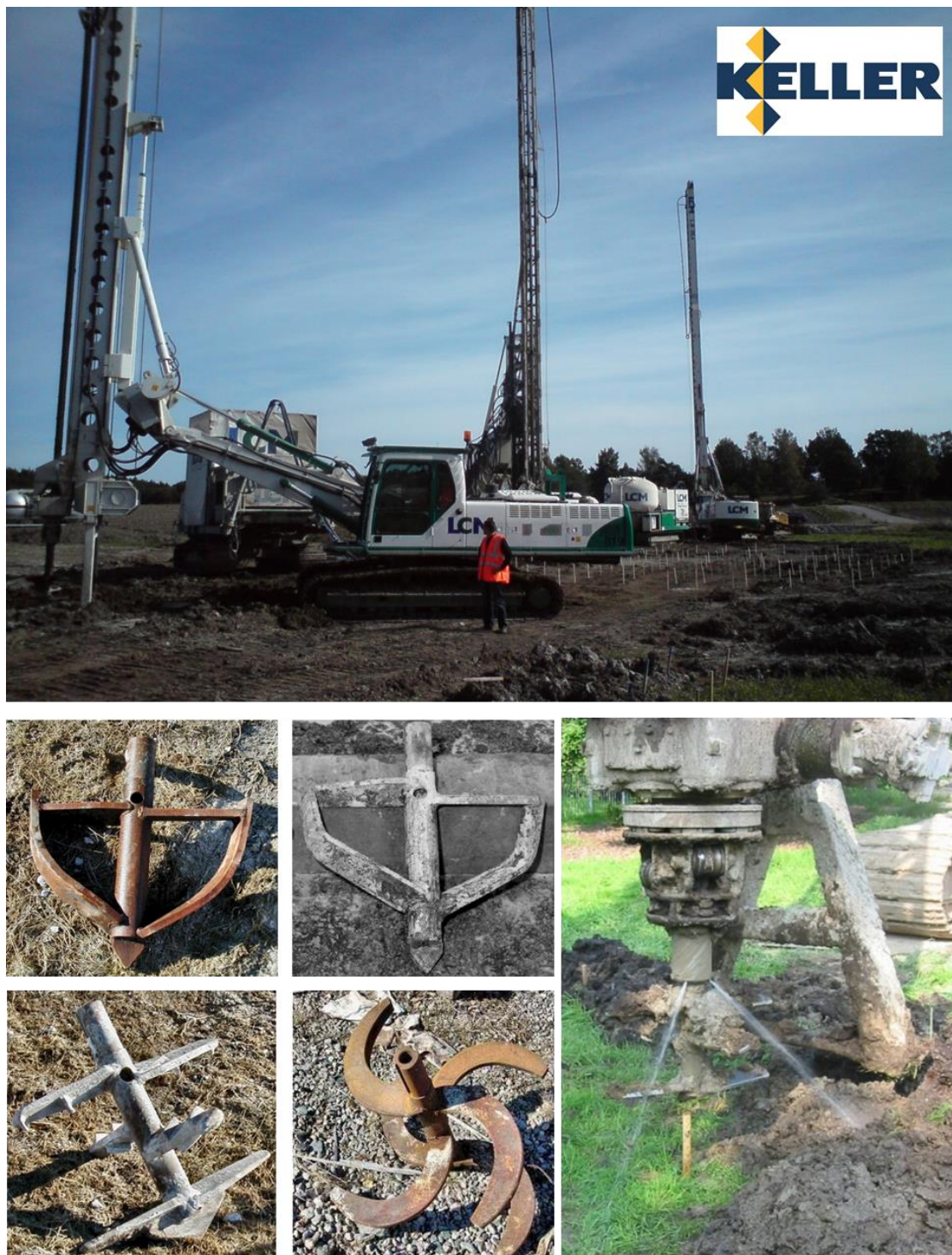
Figure 2: Illustration of the Nordic method (dry deep mixing), from Topolnicki (2012), with the courtesy of Keller
