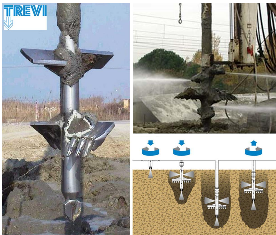
Figure 8: Trevi Turbojet technique (column diameter of 40 to 150 cm), after Topolnicki (2012) with the courtesy of Trevi
