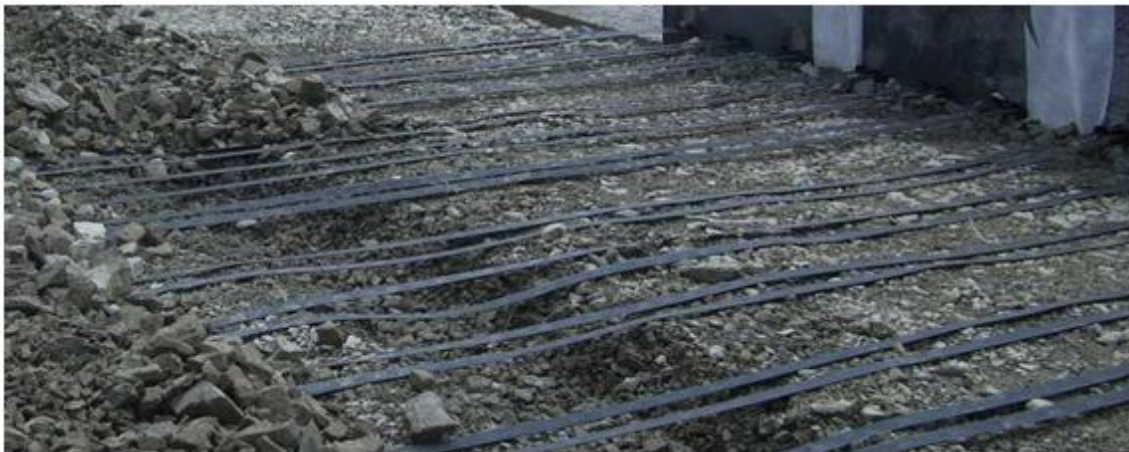
Photo 5: Extensible reinforcement, e.g. polymer strips
