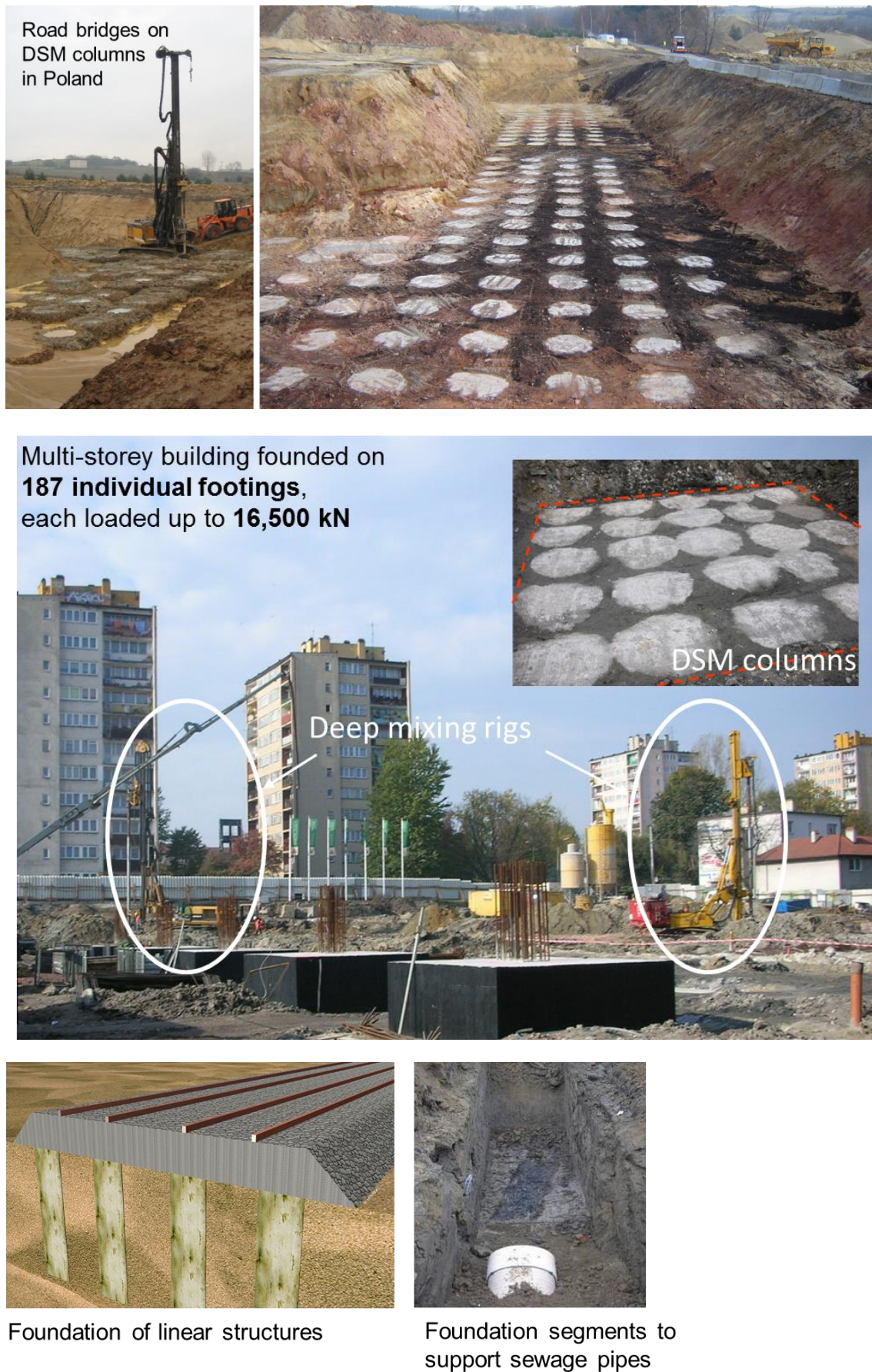
Figure 41: Examples of various structures supported by DSM elements – first part, after Topolnicki (2012) and Leemans (2012)
