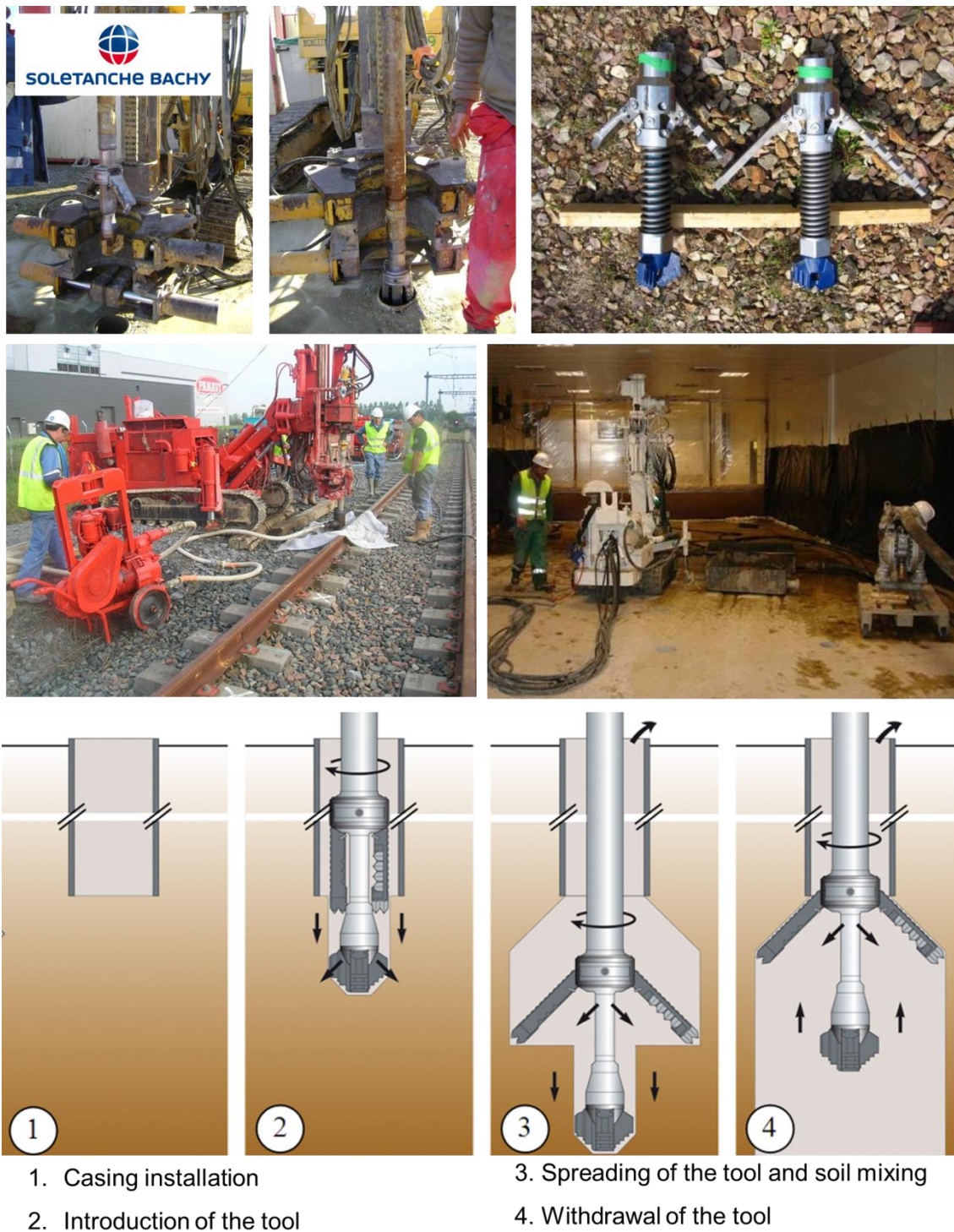
Figure 11: Soletanche Bachy wet spreadable mixing tool SPRINGSOL, from Borel (2012) and Guimond-Barrett (2012) with the courtesy of Soletanche Bachy
