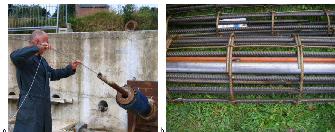
Figure 64: Examples of lost instrumentation systems integrated in a reservation tube after the installation of (a) an anchor and (b) a reinforced soil cement column, from Huybrechts (2012)
