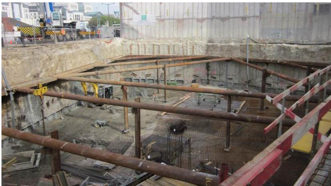
Figure 45: Shored CSM walls in Belgium, after Leemans (2012)
