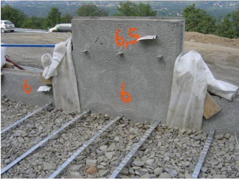
Photo 4: Inextensible reinforcement, e.g. steel strips
