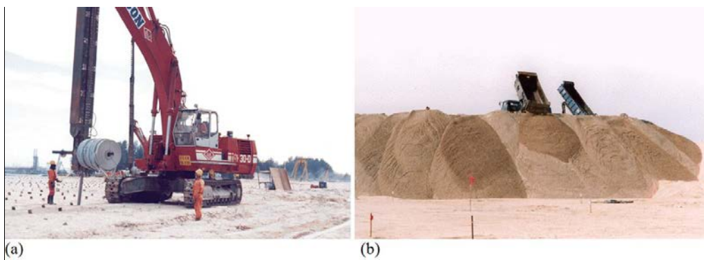
Figure 23: PVD equipment (a) and placement of preloading fill (b)
