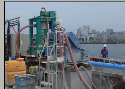
2) Re-use water as jet and soil as backfill
